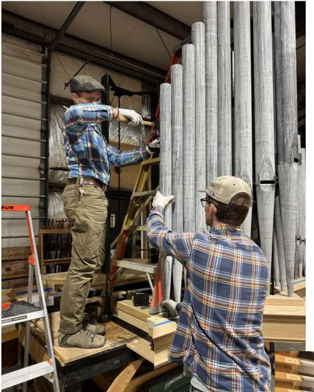
Left: Ryan (left) and Travis (right) racking (test fitting) the façade pipes. The pipes have not been washed, or buffed yet. (Travis is about six foot two inches tall), so you can see how much bigger the pipes and wooden façade will be, along with how much further the façade will stick out into the Chancel and Transept areas. Not pictured is the additional layer of the wooden façade below the working pipes.
